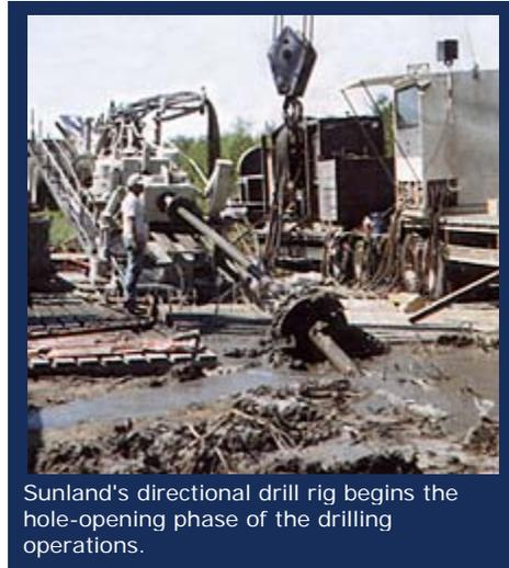
Sunland's directional drill rig begins the hole-opening phase of the drilling operations.
